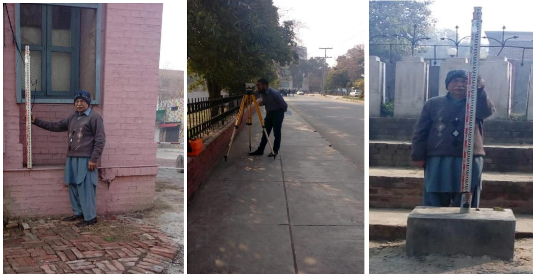
Figure 3.10 Shifting of Reduce Level from Annexe Block to Piezometers in Junaid Jamshed Cricket Stadium, UET
