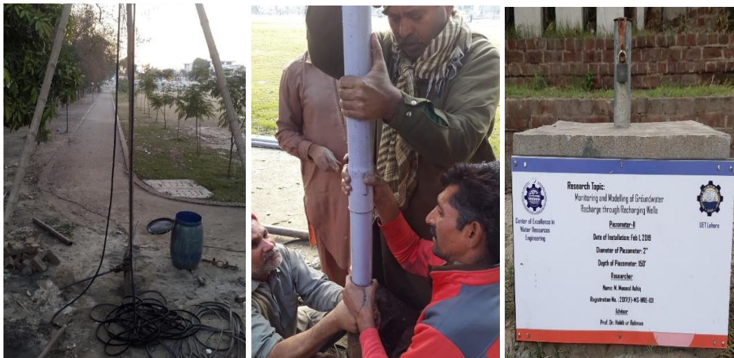
Figure 3.9 Piezometer installation in Junaid Jamshed Cricket Stadium, UET
