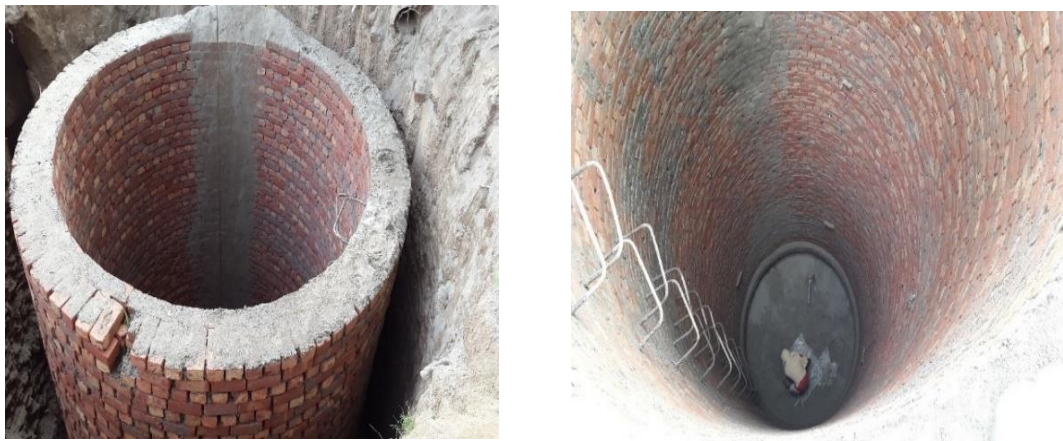
Figure 2.10 Recharging Well Wall during Construction
