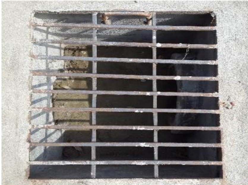
Figure 2.11 Mini Catchment Pit for Runoff Collection
