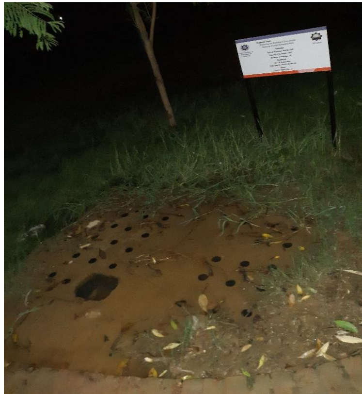
Figure 4.11 Ponding of Water on Sump connected to RW2 after Rainfall on July 25, 2019
